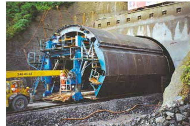
5 Innengewölbeschalung 5 Formwork for inner lining
