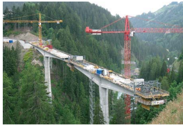
Fig. 4 Freivorbau Scuol (8. Etappe). Cantilever construction on the side Scuol (8 th segment).
