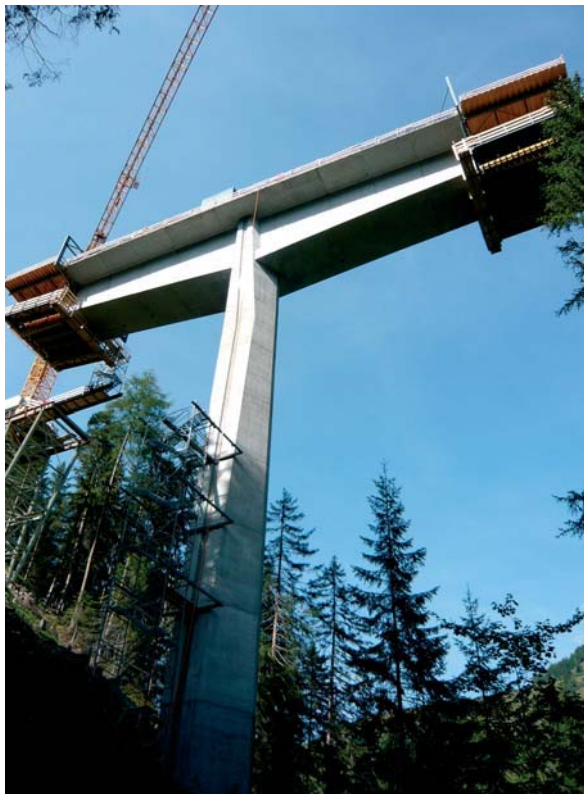
Fig. 2 Freivorbau Tarasp (4. Etappe). Cantilever construction on the side Tarasp (4 th segment).
