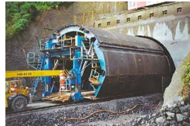
5 Innengewölbeschalung 5 Formwork for inner lining
