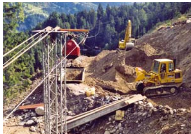
Abtransport Abtragsmaterial
